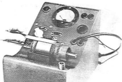
Fig. 8-8 Testing Armature Coil for Short V2187
